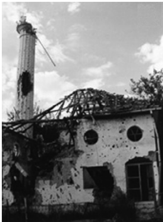
22.14. Kovačevići mosque – photo 2
