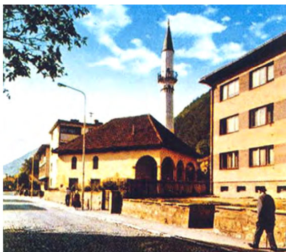
22.18. Zamlaz mosque – photo 1
