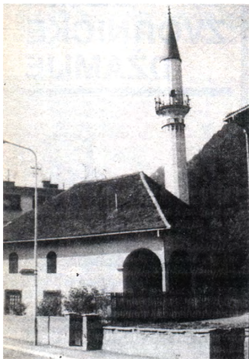
22.18. Zamlaz mosque – photo 4
